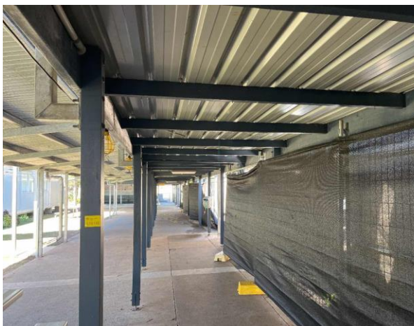
Line ID 45: External, Walkways, Throughout, Timber to Cover, Blue (Dark) Paint - Lead Detected (<0.005% w/w)
