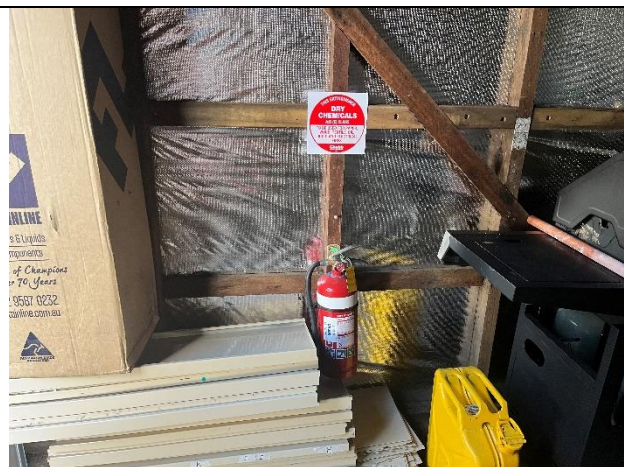
Photo 04. Fire Extinguisher adjacent chemical storage in the Building D Mower shed.
