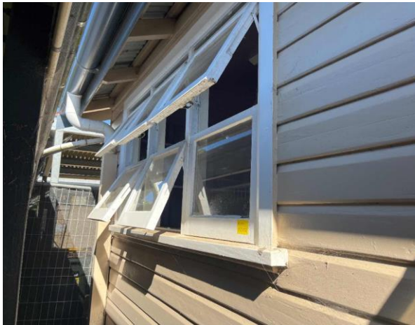
Line ID 7: External, Building E, Throughout, Wooden Windows, Window Caulking - No Asbestos Detected
