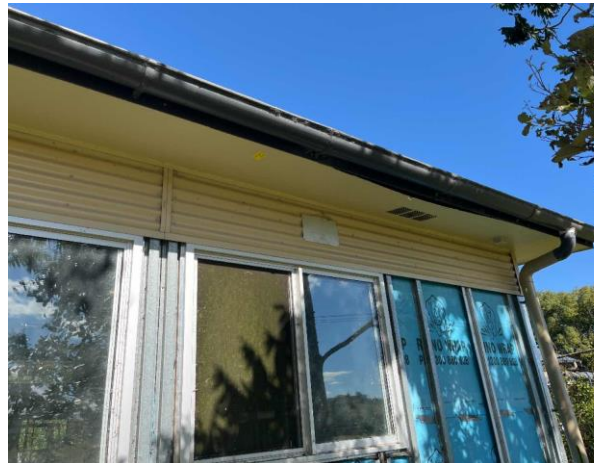
Line ID 14: External, Building I, Throughout, Eaves, Fibre Cement Sheet - No Asbestos Detected
