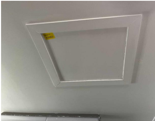
Line ID 31: Internal, Building J, Boys Toilet, Man Hole Cover, Fibre Cement Sheet - No Asbestos Detected
