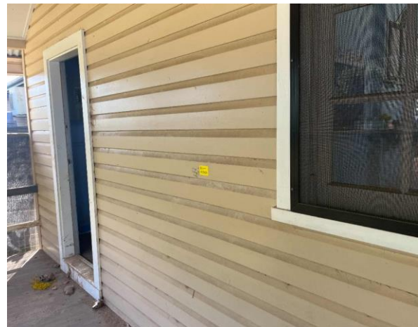
Line ID 10: External, Building F, Throughout, Walls, Cream Paint - No Asbestos Detected
