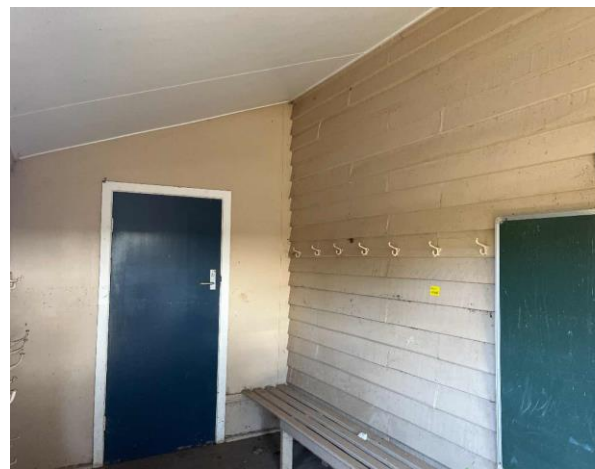
Line ID 6: External, Building E, Throughout, Walls, Beige Paint - No Asbestos Detected
