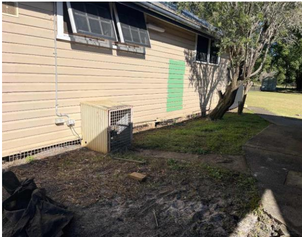
Line ID 74: External, Building F, Subfloor – No Access
