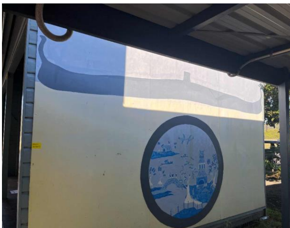
Line ID 11: External, Building G, Throughout, Wall, Fibre Cement Sheet - No Asbestos Detected
