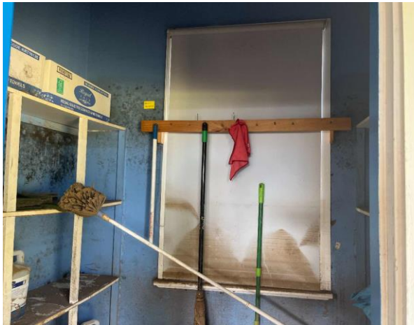
Line ID 28: Internal, Building F, Southwest Storeroom, Walls, Compressed Cement Sheet - No Asbestos Detected
