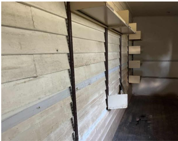
Line ID 24: Internal, Building E, Western Room, Walls, Beige Paint - No Asbestos Detected
