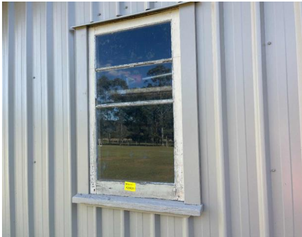
Line ID 3: External, Building D, Eastern Wall, Wooden Framed Window, Window Caulking - No Asbestos Detected
