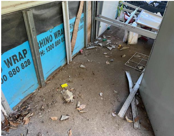
Line ID 13: External, Building I, Throughout, Debris, Compressed Cement Sheet - No Asbestos Detected
