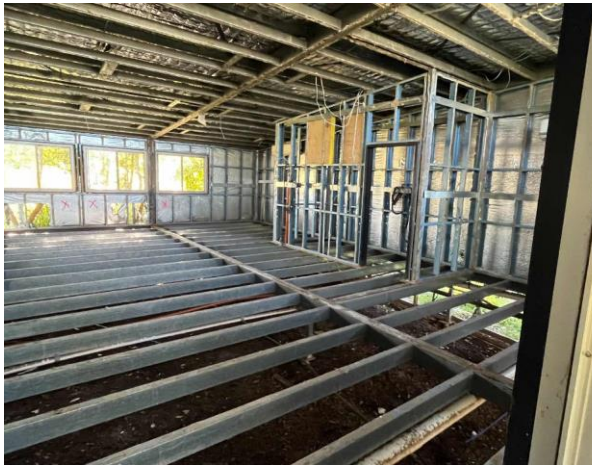
Line ID 66: Internal, Building I, Throughout, Walls and Ceiling, Sarking Insulation - Suspected SMF
