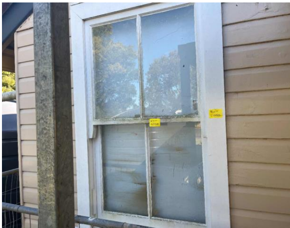
Line ID 9: External, Building F, South Side, Window Frame, Window Caulking - No Asbestos Detected
