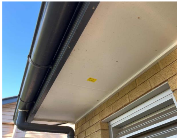
Line ID 16: External, Building J, Throughout, Eaves, Fibre Cement Sheet - No Asbestos Detected
