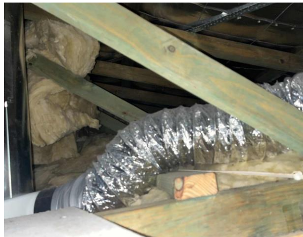
Line ID 69: Internal, Building J, Throughout, Flexible Ductwork, Internal Insulation - Suspected SMF
