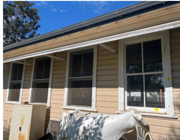
Line ID 2: External, Building A, Throughout, Wooden Framed Windows, Window Caulking - No Asbestos Detected
