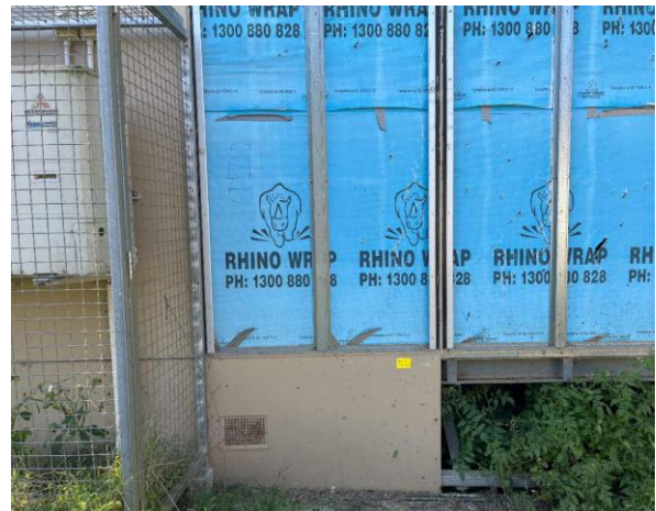
Line ID 44: External, Building I, Throughout, Walls, Beige Paint - Lead Detected (<0.005% w/w)
