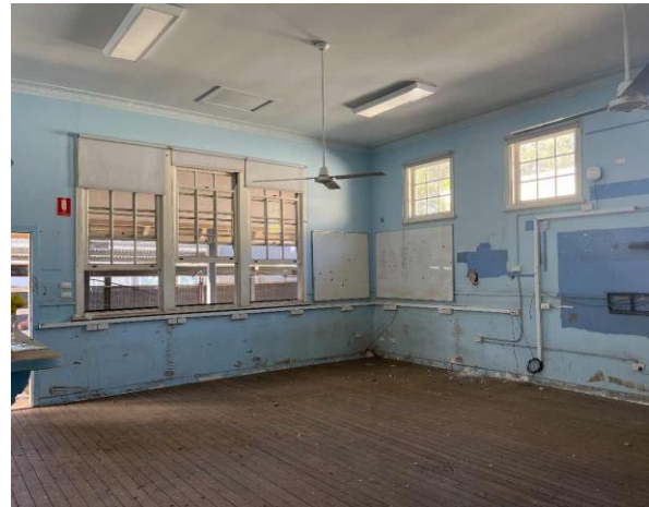
Line ID 76: Internal, Building F, Ceiling Void – No Access
