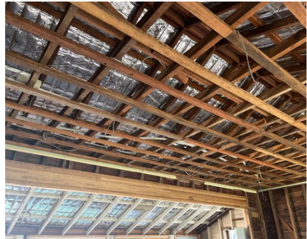
Line ID 61: Internal, Building A, Throughout, Ceiling, Sarking Insulation - Suspected SMF
